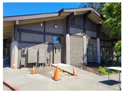
...For The Building's Heating and Cooling Equipment (HVAC) The old, weather-worn enclosure encircling the HVAC equipment on the east side of the building has been removed and is being replaced with a slightly expanded enclosure to include the emergency generator we added three years ago.
